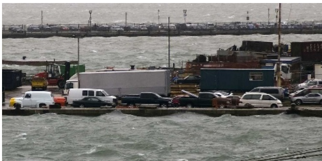
Figure 11. Waves overtop the quay wall at Southampton Docks at high tide on 10 March 2008 (Source: Barry Marsh, School of Ocean and Earth Science, University of Southampton)
